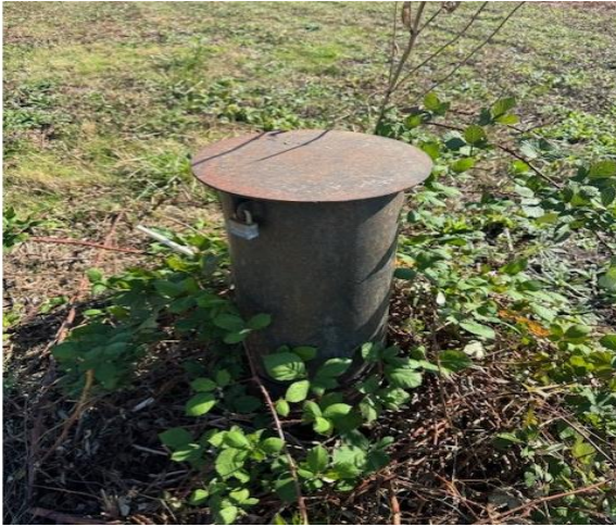
Figure 2: Test Well 1 at 5440 SW 6 th Avenue
