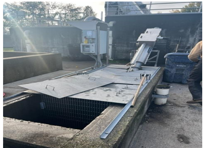
Fig. 10 Septage Receiving Station
