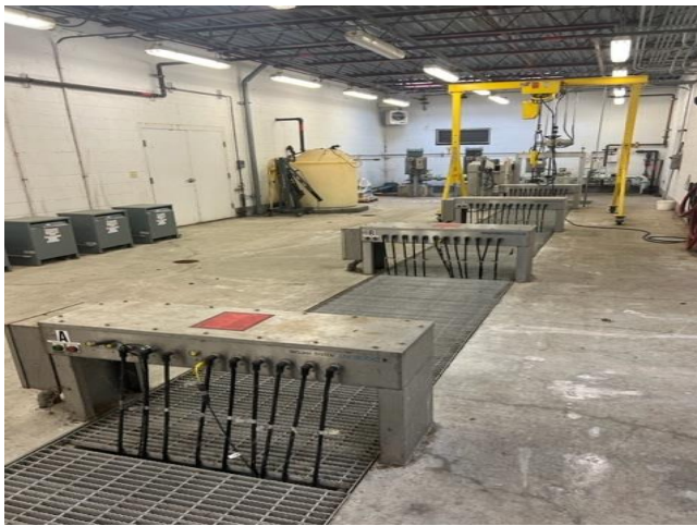
Fig. 9 Ultraviolet (UV) Bank
