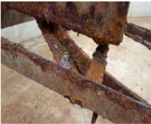
Figures 3-5: Corroded Metal in Primary Clarifier Basin
