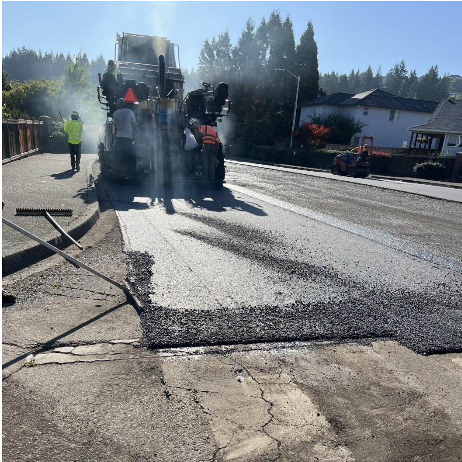
New Wearing Surface placed in Two Lifts
