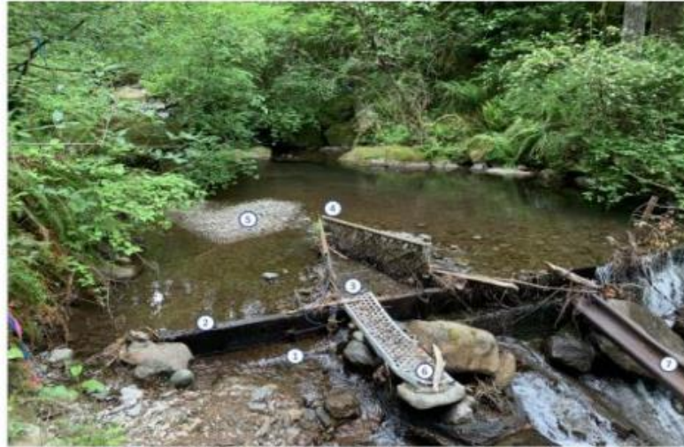
Figure 1: Photo of existing dam and intake structure from downstream of dam looking upstream
