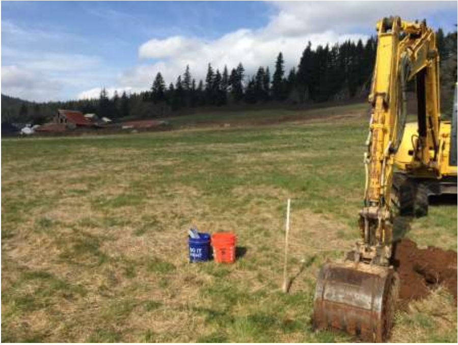
Test Pit TP-9
