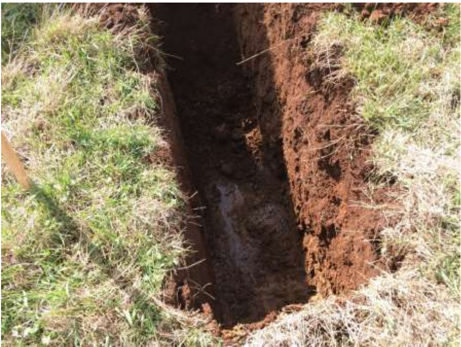
Test Pit TP-7
