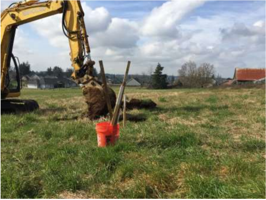
Test Pit TP-7
