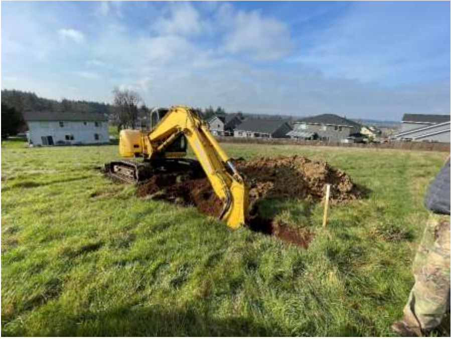
Test Pit TP-3
