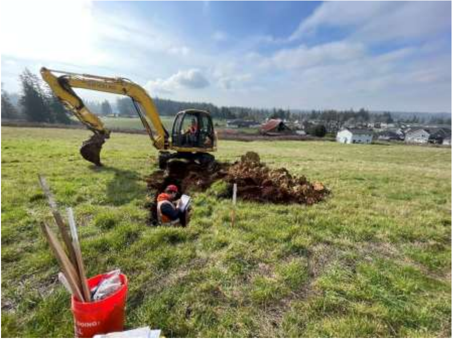
Test Pit TP-4
