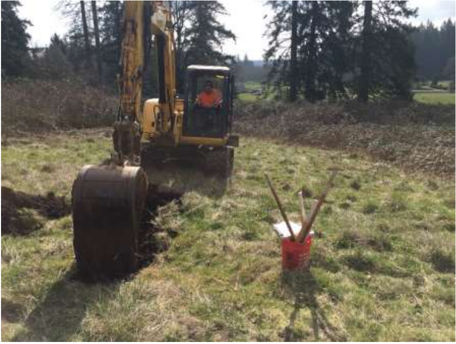
Test Pit TP-8
