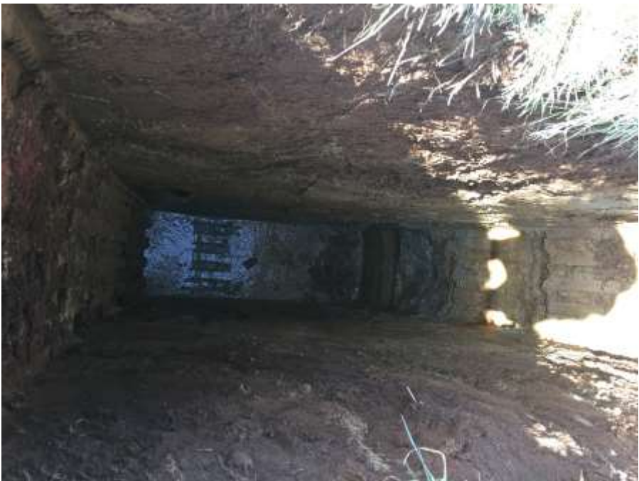
Test Pit TP-9
