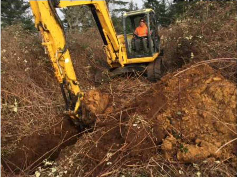
Excavator Test Pits
