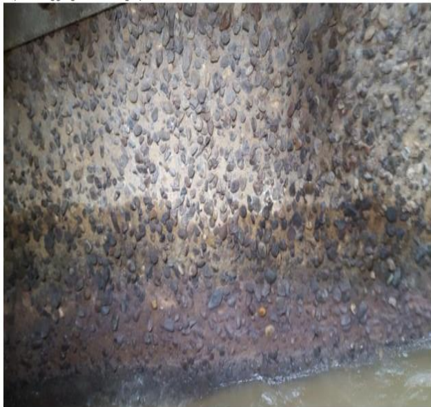
Figures 1-2: Damaged concrete in Headworks
