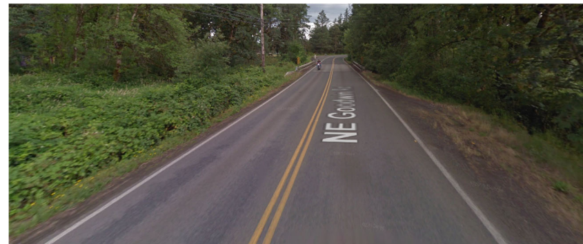
Figure 14. Northbound NE Goodwin Rd near Camp Lacamas
