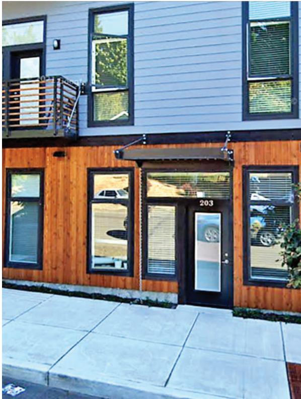
Figure 64. Example of Walkup Frontage
