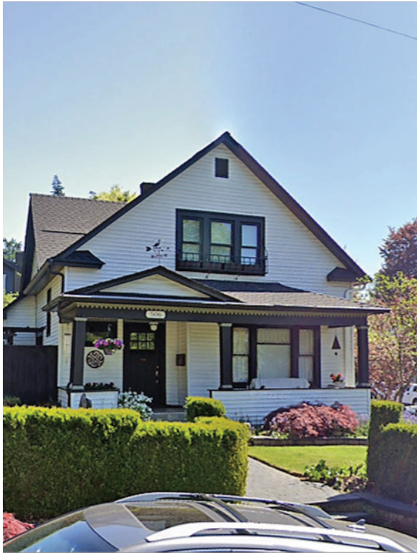
Figure 52. Example of Porch Frontage
