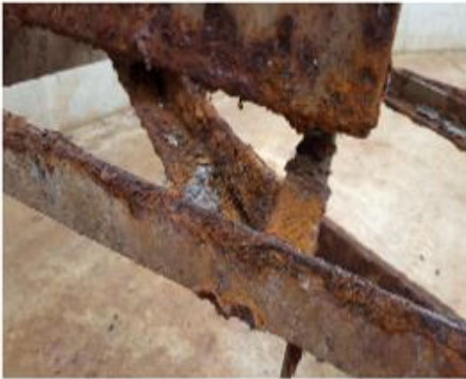
Figures 3-5: Corroded Metal in Primary Clarifier Basin
