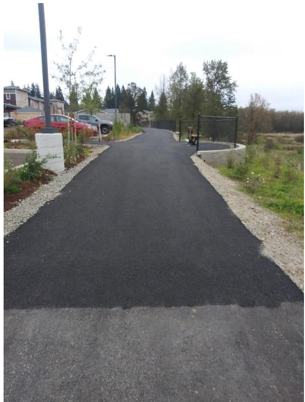
Figure 2: Regional Trail overlook with park bench.
