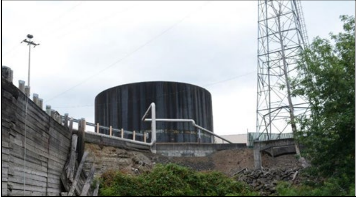
Photograph 9. Aboveground storage tank, a 40,000-gallon steel oil tank that has been previously cleaned and disconnected.
