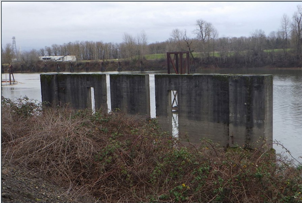
Photograph 6. Concrete footing from the Berger Crane gantry.
