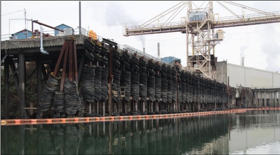
Photograph 5. The PECO Dock, supported by approximately 400 wood piles.
