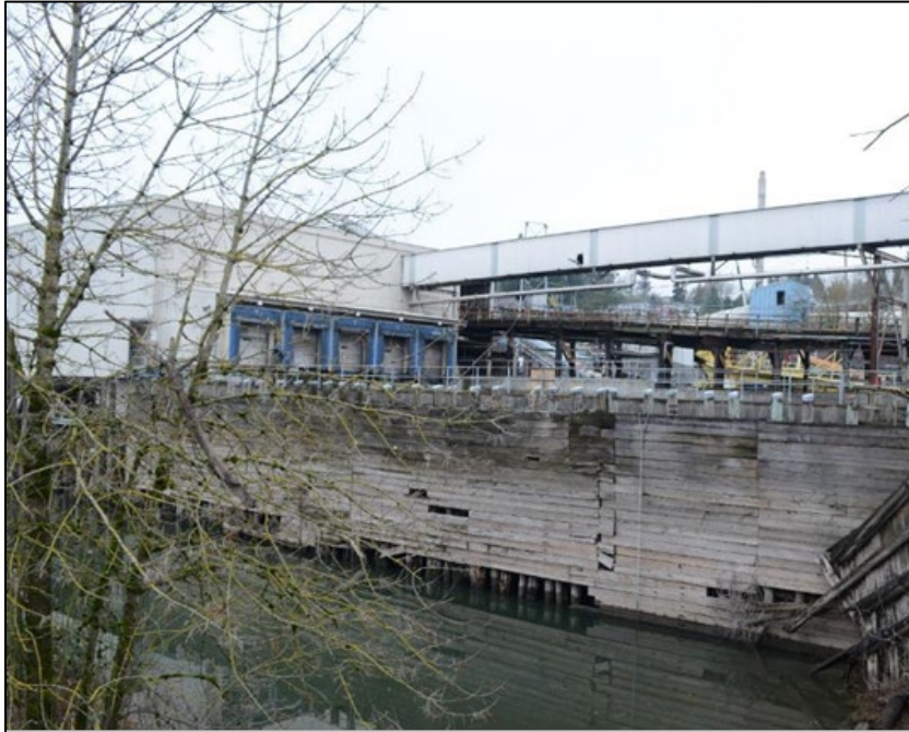
Photograph 1. Truck Dock which is supported by approximately 220 pilings constructed from wood and pipe.
