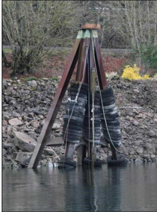
Photograph 7. Typical HP pile dolphin with tire bumpers attached.
