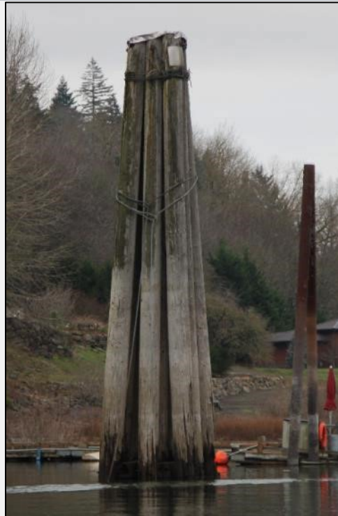
Photograph 8. Typical timber head dolphin.
