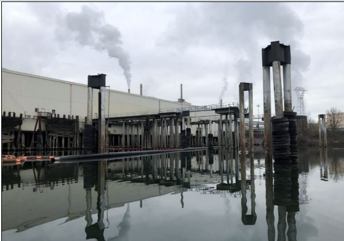
Photograph 4. Three piers extend from the Dock Warehouse that are supported by 54 concrete piles along with 21 carbon steel pipe piles. Three guidance dolphins are arranged at the end of the piers.
