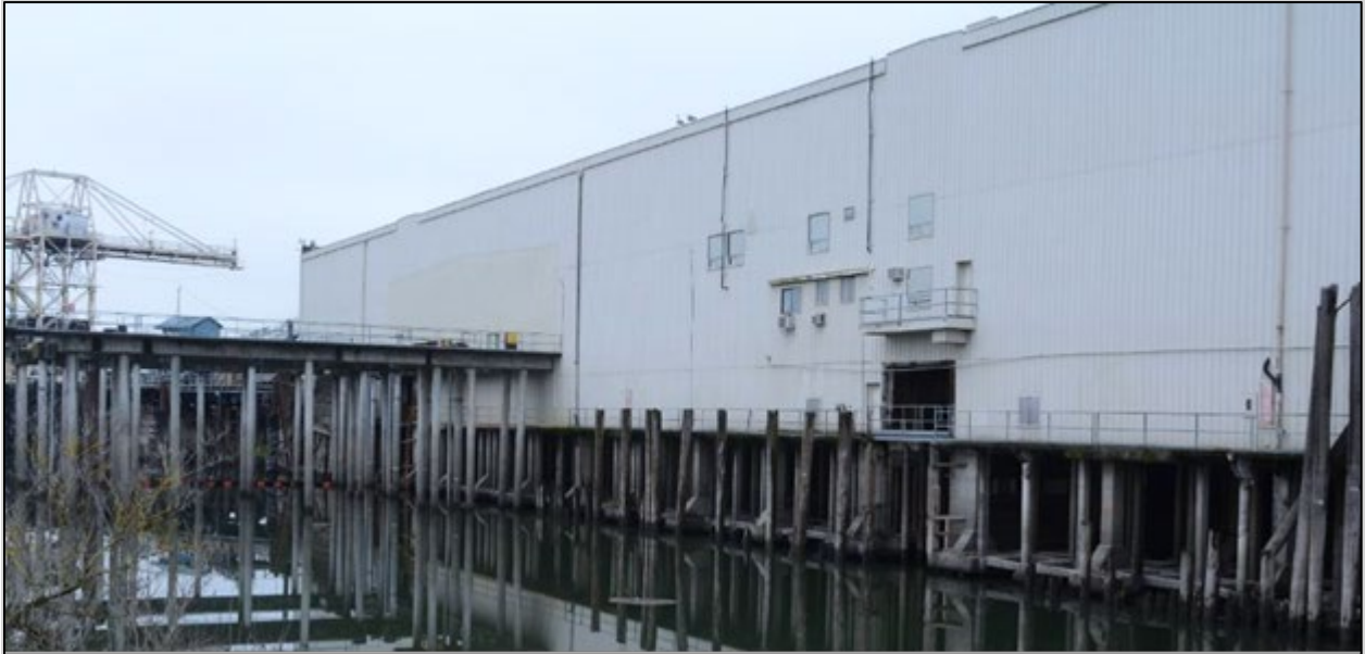
Photograph 3. Dock Warehouse situated between the Truck Dock and PECO Dock and supported by approximately 800 piles, with foundations on the riverbank side.
