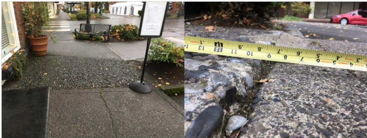
Exposed Aggregate Sidewalk Panels Downtown
