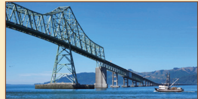
The Astoria-Megler Bridge linking Oregon to Washington State
