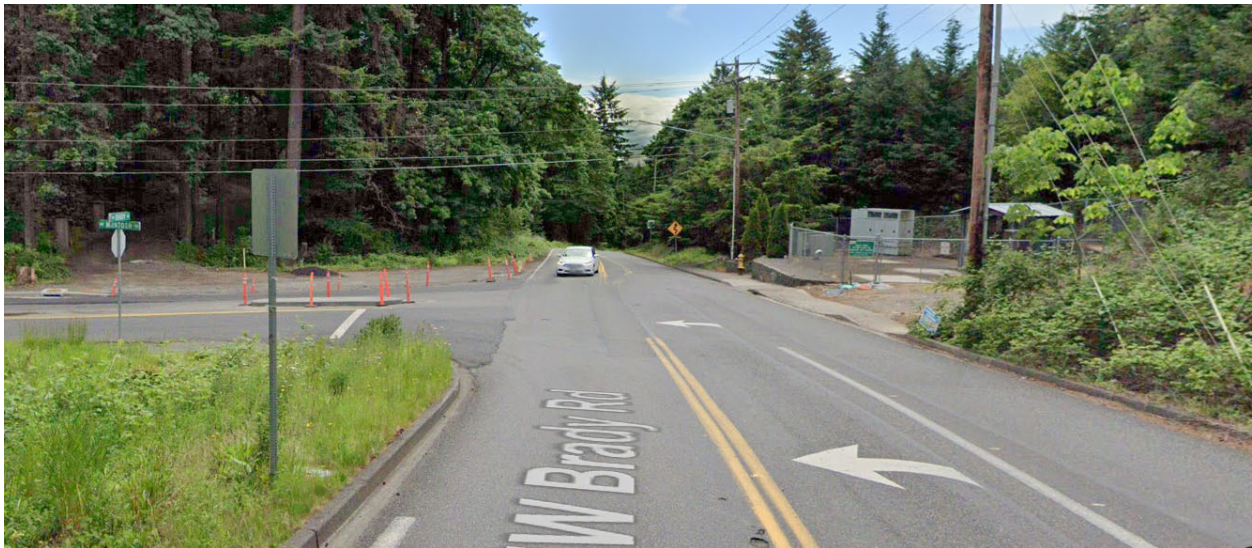
Figure 3- Left-Turn Lane at the Intersection of McIntosh Rd and Brady Rd Provides a Safe Turning Movements
