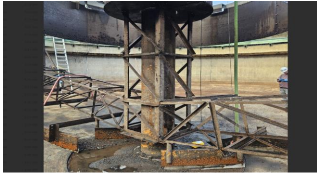
Figure 2-4: Clarifier Arm Damage
