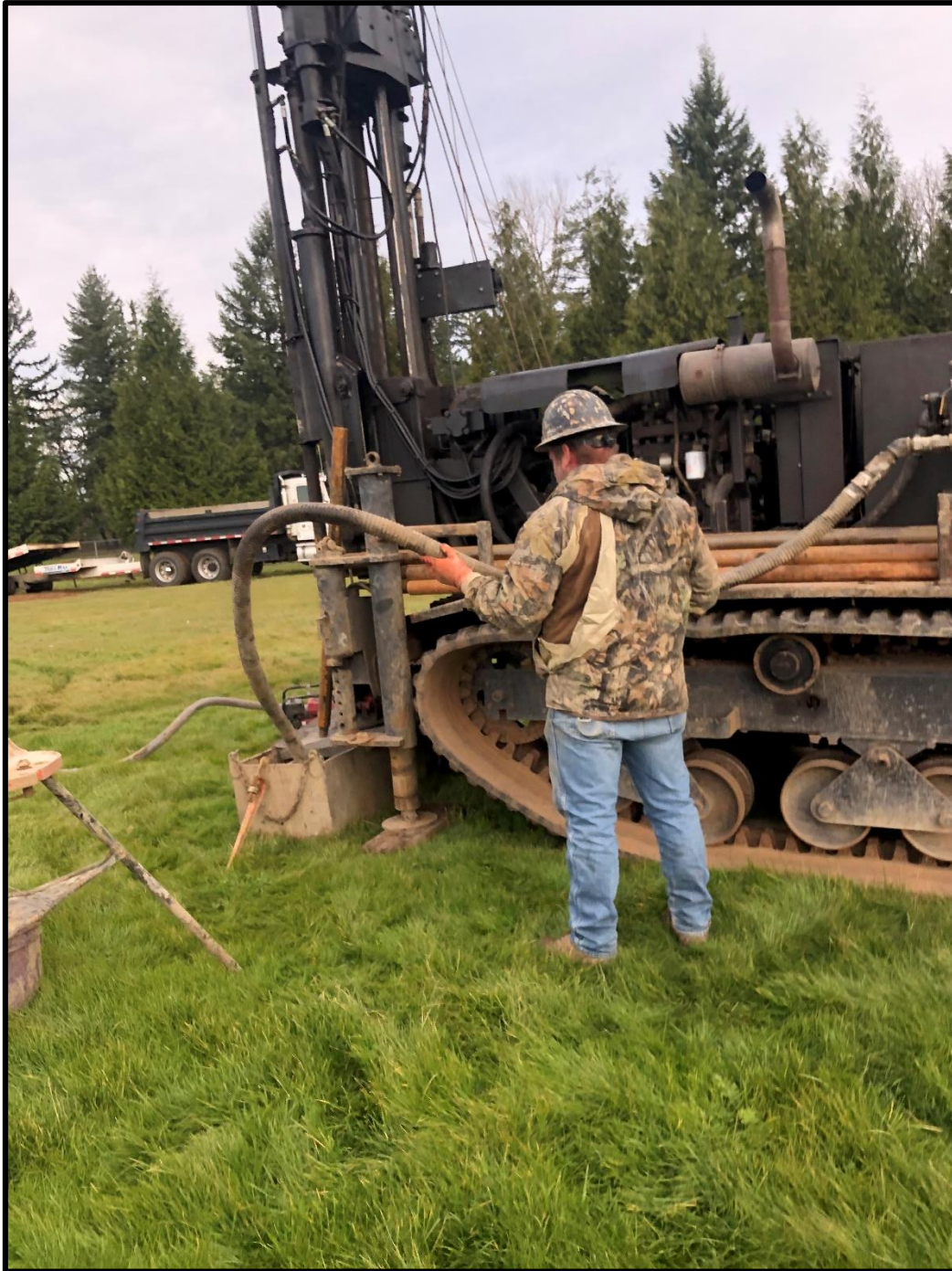
Soil Boring, SB-1
