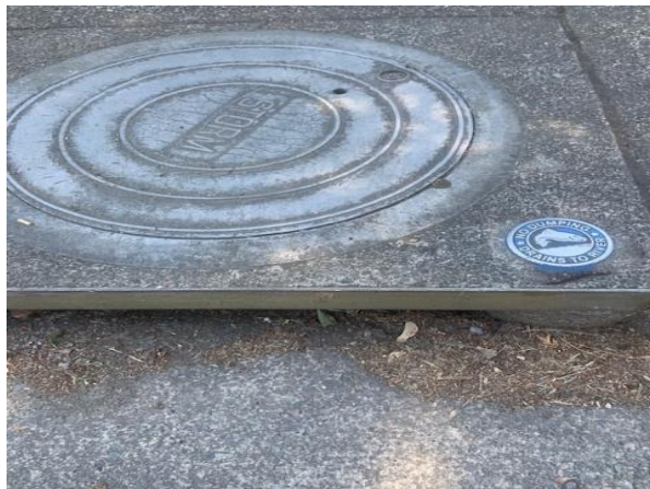
Figure 1: Curb inlet with Camas medallion
