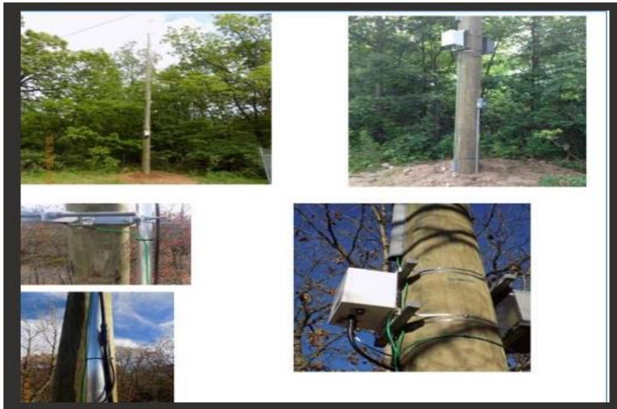
Figure 1: Example of Utility Poles with Data Collectors
