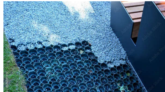
Permeable surfaces should be used in the overall stormwater management plan for developments (Source: © Michal / Adobe Stock)
