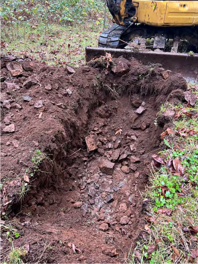
I-7. Bedrock @ 2.5 ft. bgs
