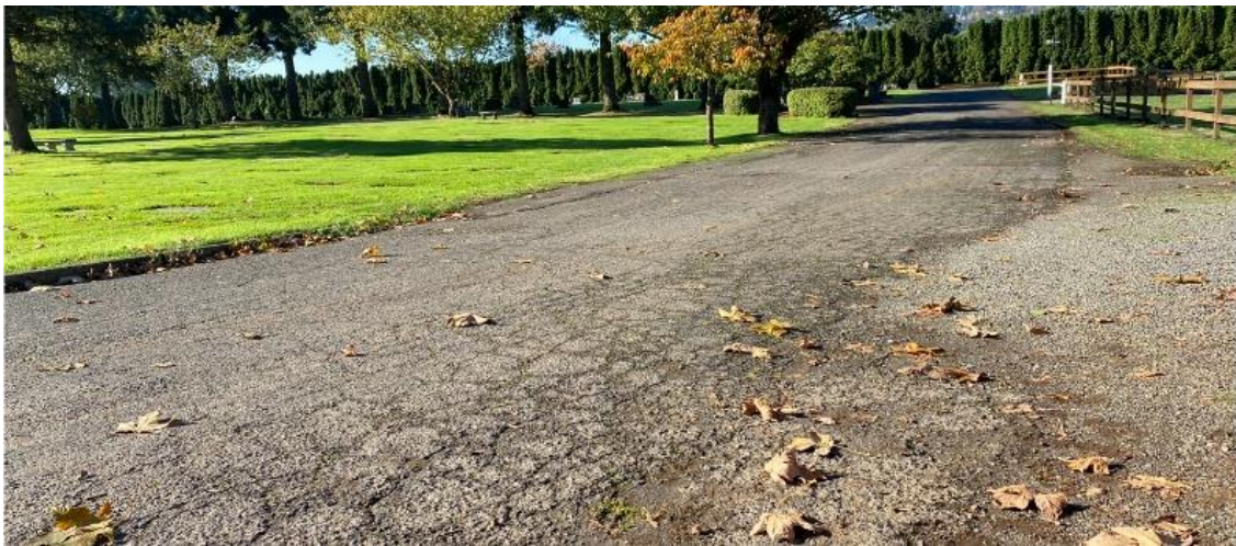
Pavement Condition Sample
