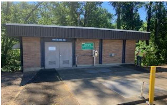
Fig.5: Front of Pump Station
