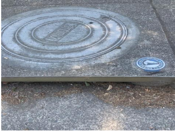
Figure 1: Curb inlet with Camas medallion
