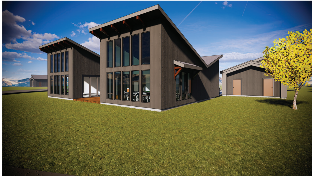
SIDING TO BE 4" VERTICAL CEDAR STAINED SMOKE GRAY
