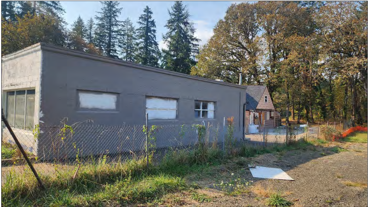
Photo 3. Southeast side of the study area at NE Everett Street facing offsite to the southwest.
