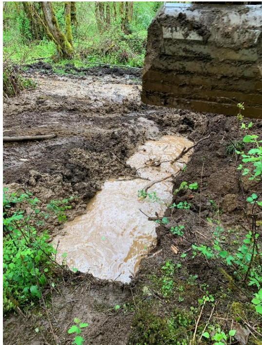
Photo 2. Seepage ponding at TP-2 during backfill operations.
