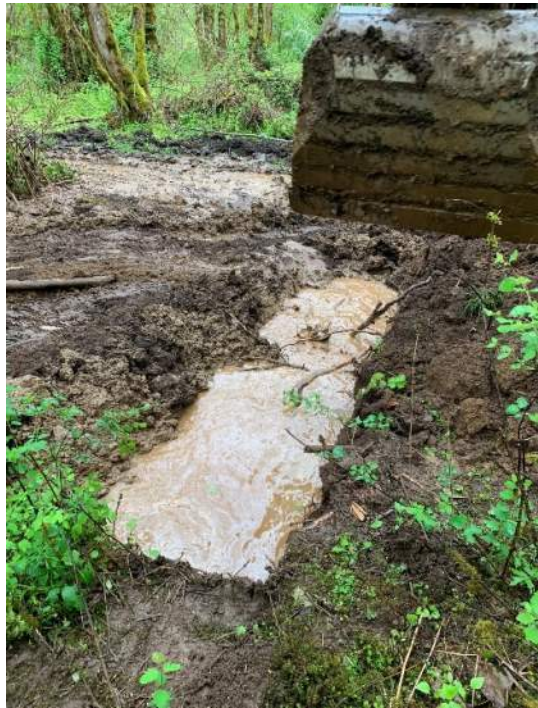
Photo 2. Seepage ponding at TP-2 during backfill operations.
