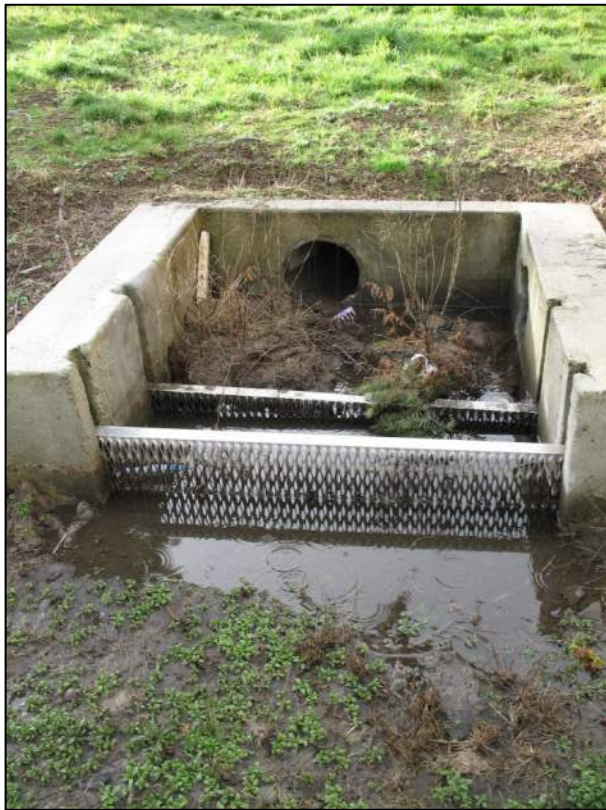
Sediment Trap with Accumulated Sediment
