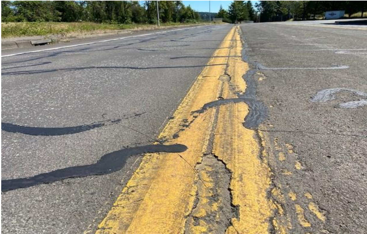
NW Parker Looking South towards WaferTech: Layers of existing street markings were delaminating from the pavement surface.
