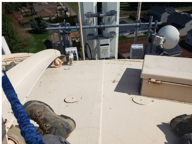
Conduit penetration adjacent ladder at edge.
