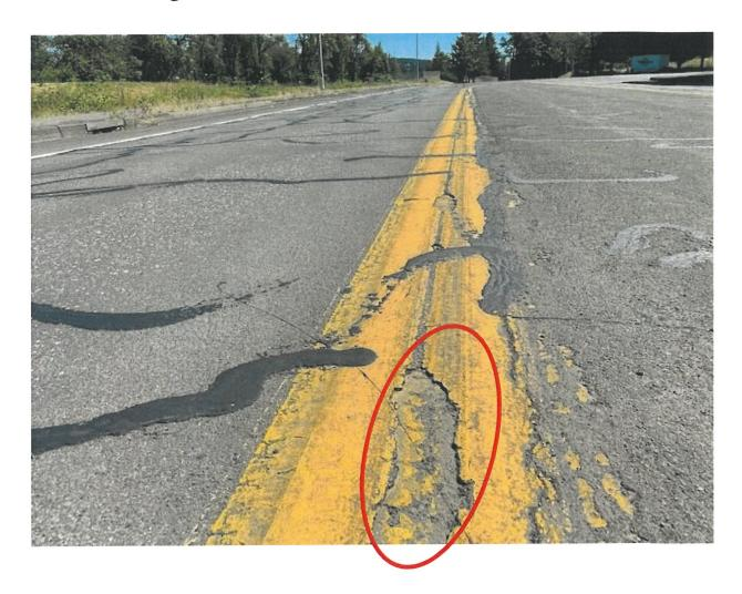
Existing Pavement Markings consisted of layers of thermo-plastic and paint. These markings were required to be removed by a hydro-blasting truck to ensure the new Slurry Seal surfacing would bond to the existing roadway.
