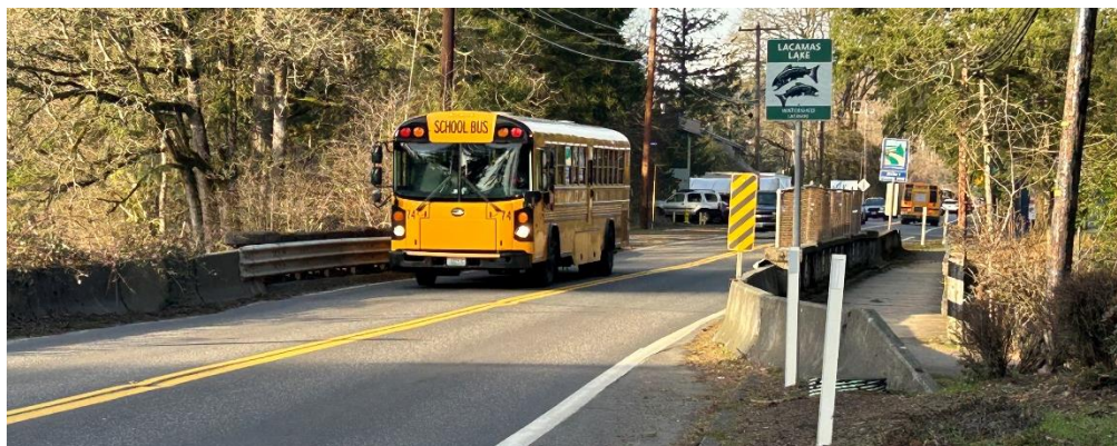
Existing SR500 (Everett Street) Lacamas Lake Bridge
