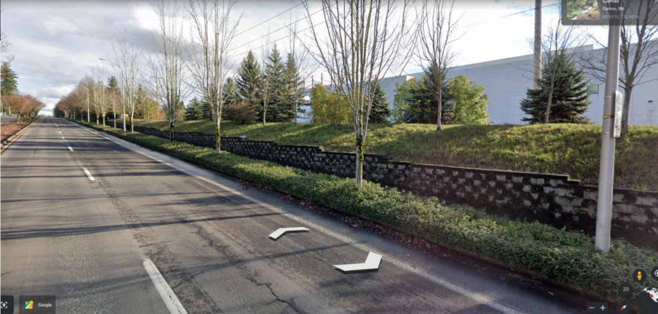
Looking EAST on NW Lake Road
