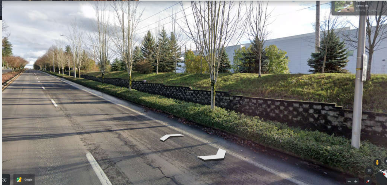
Looking East on NW Lake Road →
