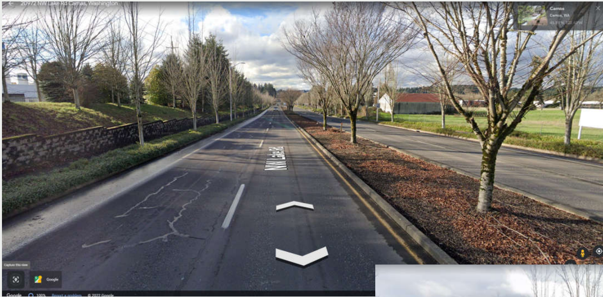
← Looking West on NW Lake Road
