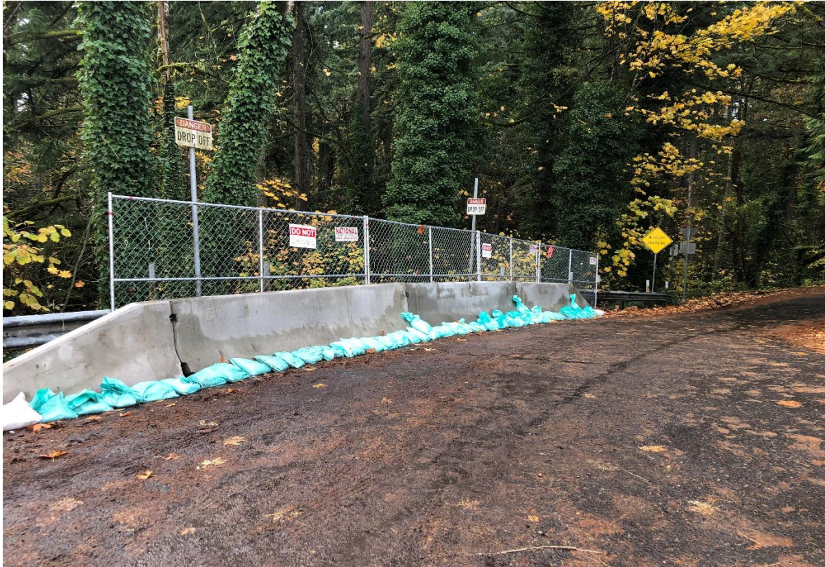
Photo of the Ostenson Canyon Winterization Measures
