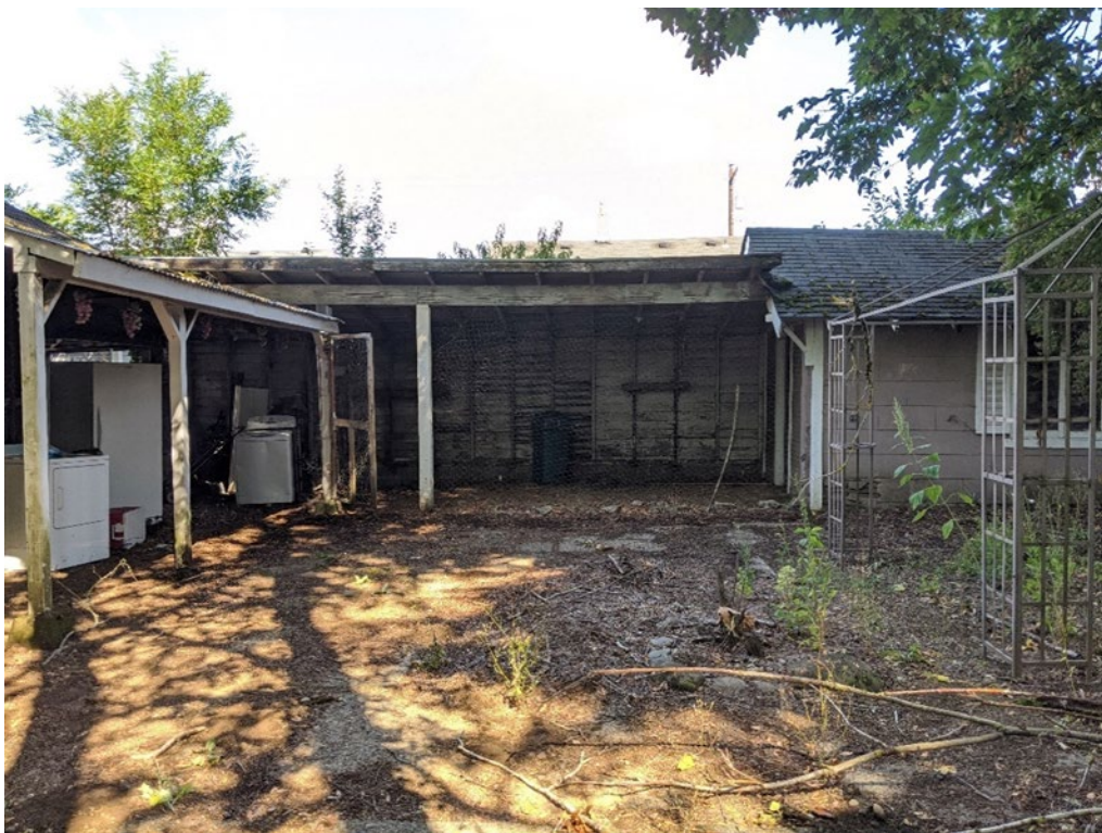
Figure 12. View of outbuildings, facing west.
