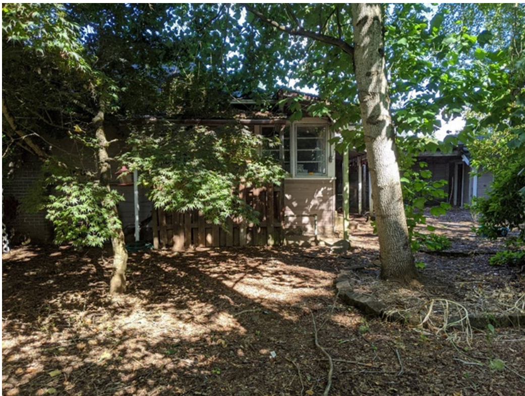
Figure 10. View of single-family residence, facing north.
