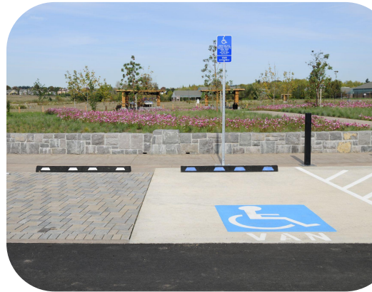
ADA Accessible Parking
