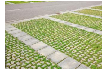
Driveways using permeable pavers
