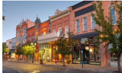
Weather protection and landscaped bollards support a pedestrian friendly streetscape (Source: © SeanPavonePhoto/ Adobe Stock)
