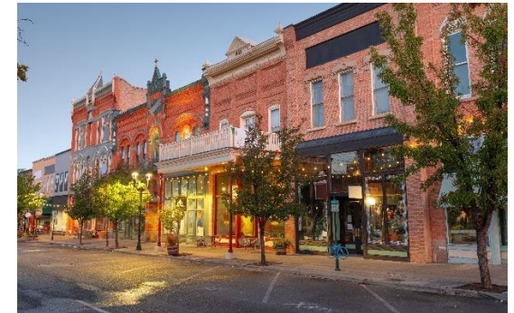
Weather protection and landscaped bollards support a pedestrian friendly streetscape (Source: @ SeanVavonePhoto / Adobe Stock)
