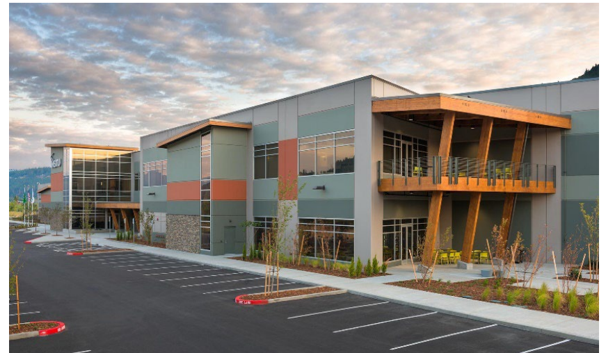
The LEED Silver In-situ Building in Bingen, OR, reflects the Pacific Northwest style, including wood siding and drought tolerant landscaping. (Source: lewisbuilds.com/projects/insitu)
