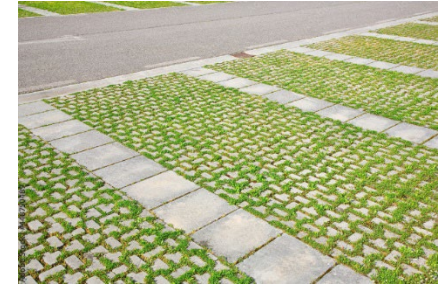
Driveways using permeable pavers (Source: © Francesco Scatena/ Adobe Stock)
