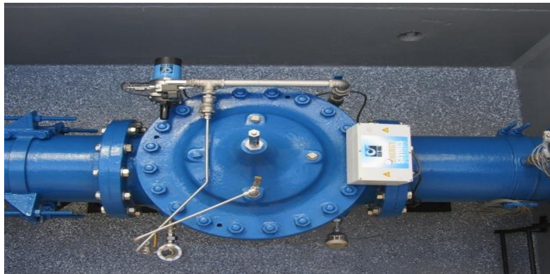
Figure 1: PRV Valve
