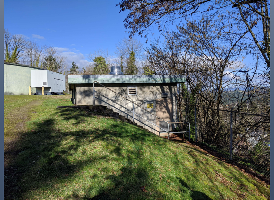
BOOSTER PUMP STATION
