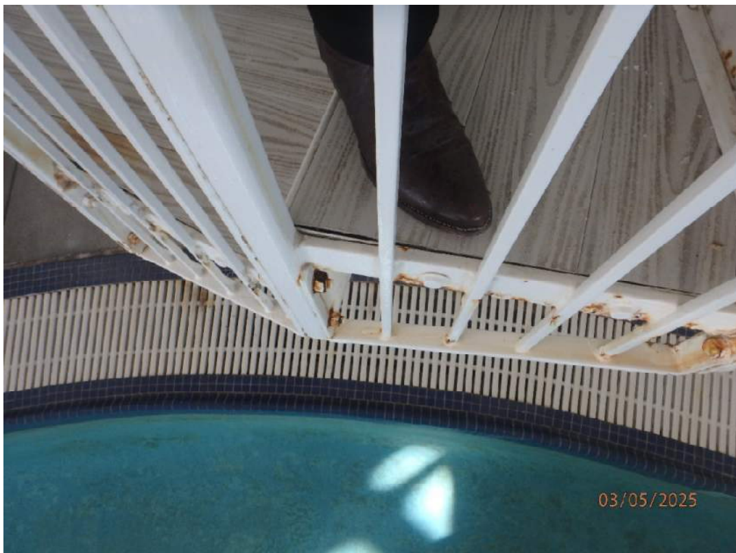
Figure 5: Typical Bolts at Spiral Guardrails
