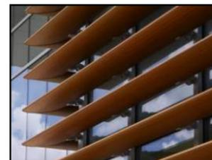
ALUMINUM SHADING DEVICE
