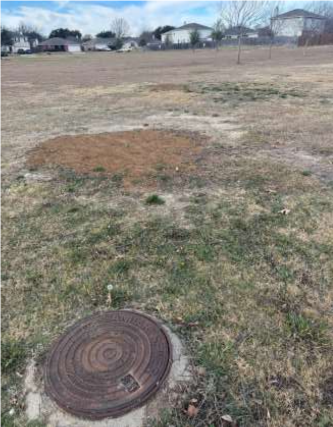
Existing site conditions showing SS line and removed trees 1/13/26
