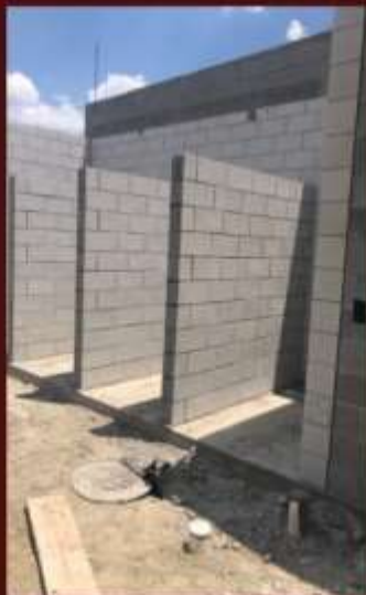
KENNELS BEING BUILT
