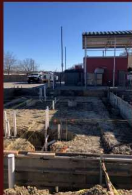
ROOM STRING LINES
