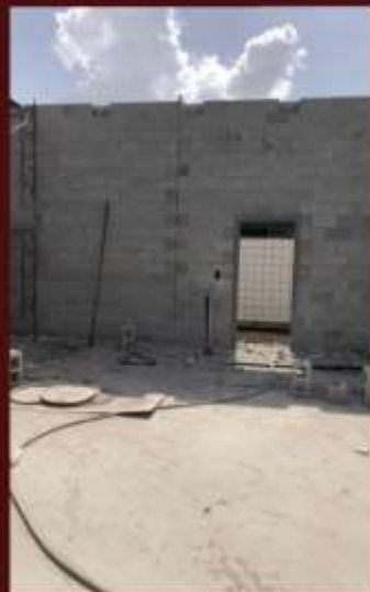
CMU BLOCK GOING UP
