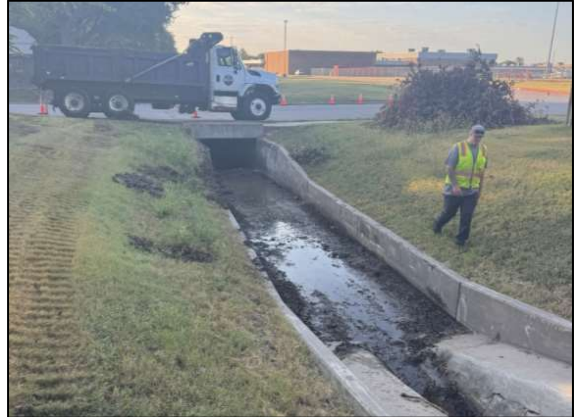
Public Works removed sediment to restore drainage.
