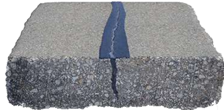
Crack Seal application
