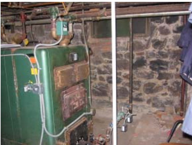
Fig 29: Basement - Cut stone masonry walls
