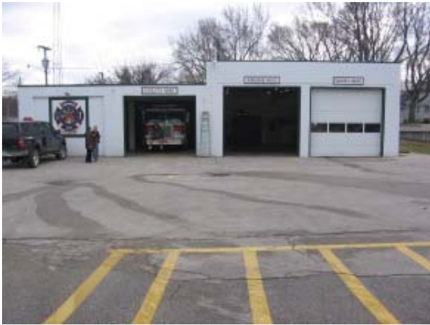
Fig 65: Garage- North elevation
