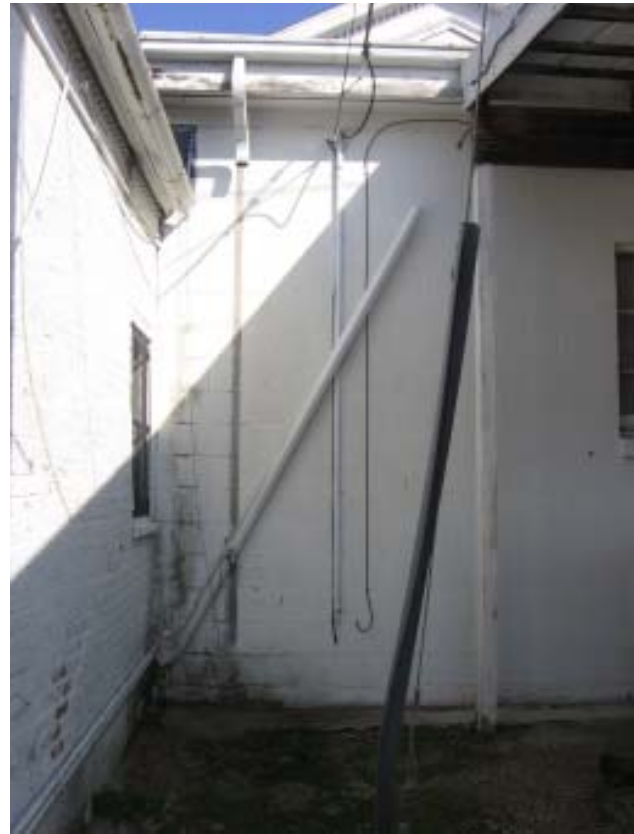
Fig 13: South elevation - Downspouts at corner of 1949 Addition and Jail
