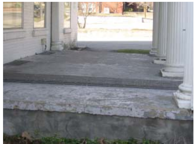
Fig 5: Concrete slab of north porch
