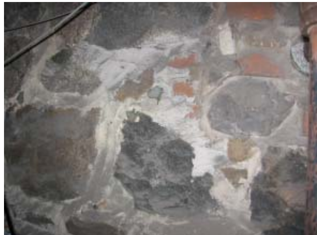
Fig 30: Basement - Cut stone masonry walls repointed
