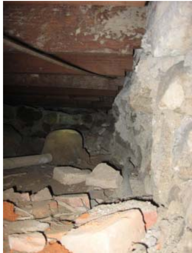
Fig 45: First Floor Structure - Notched joists at east bearing in west wing
