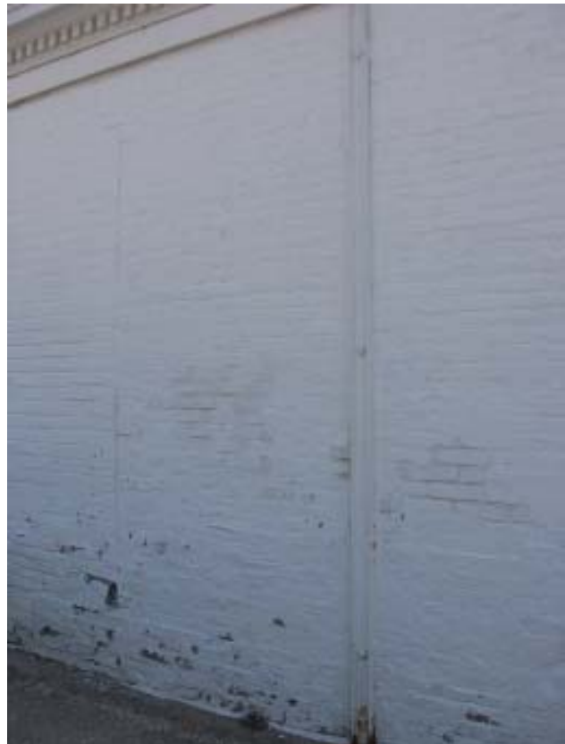
Fig 25: West elevation - Existing channel brace
