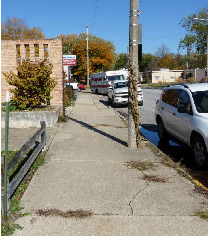
Main St. North
