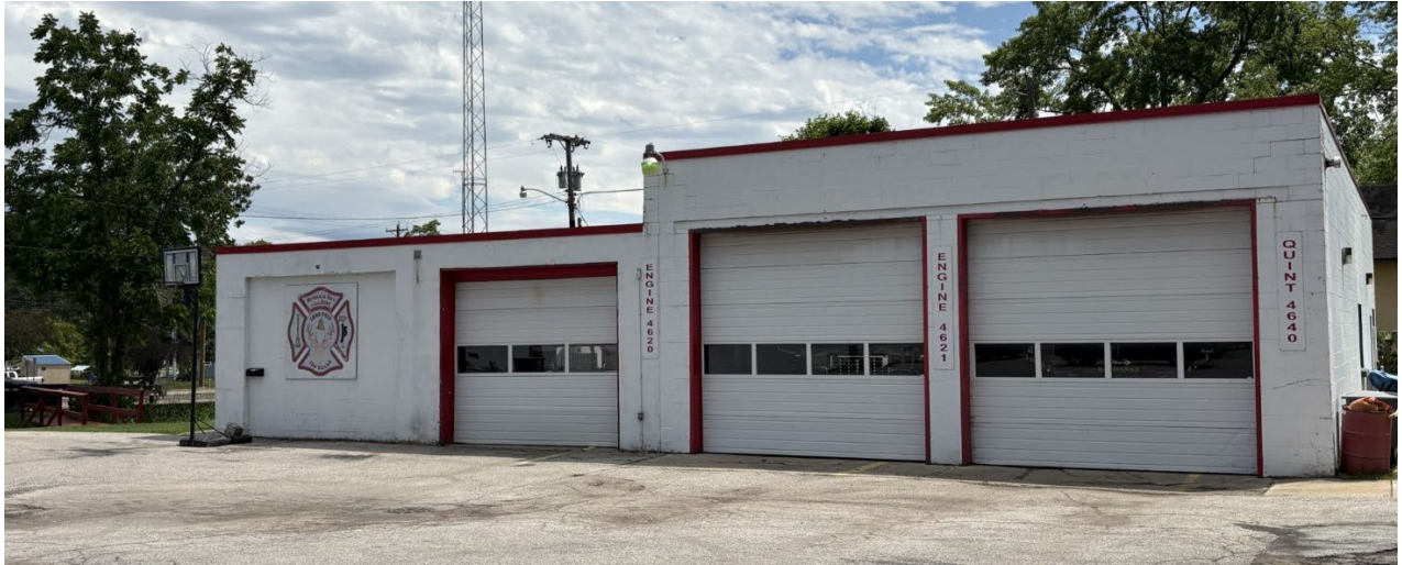
View looking south from W Front Street.
