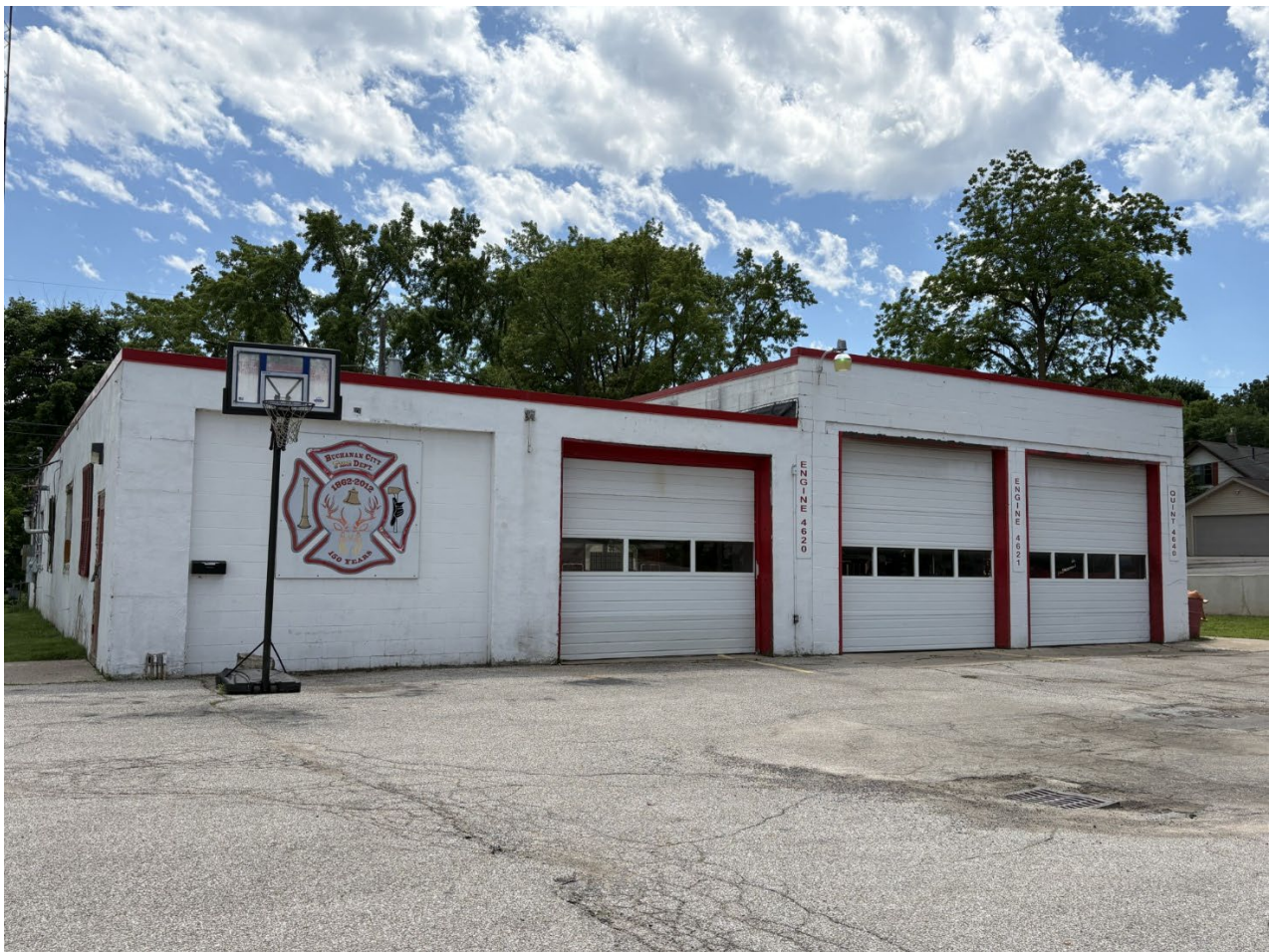
View looking southwest from parking lot
